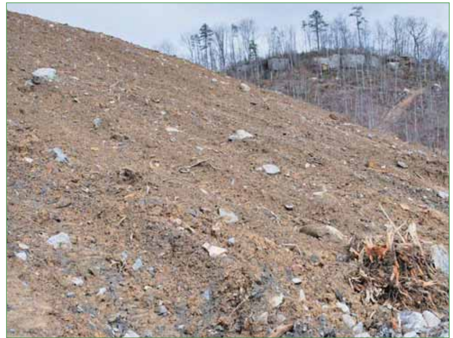
This will be the typical appearance after grading -- loosely distributed rock and organic material.
